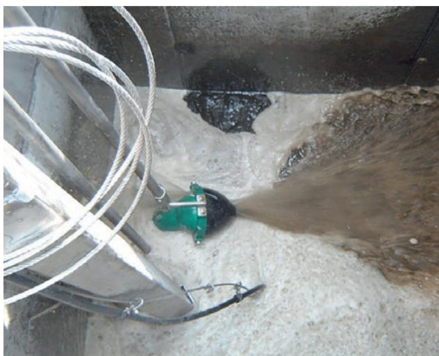
Rührdüse in Betrieb | Agitating nozzle in operation
